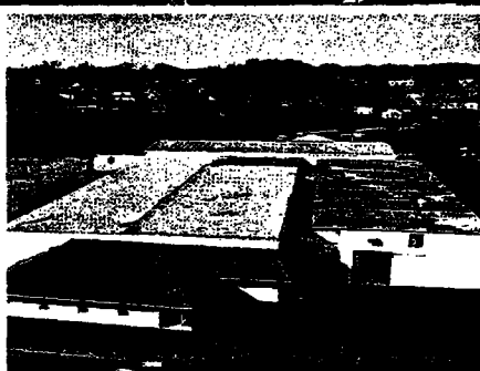
The plant in the USA is located at Anderson, South Carolina and it is completely geared for the manufacture of pipe-seals for the American market.
