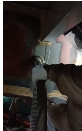
Vacuum blast at weld seam, erection joint, pipe joint, etc
