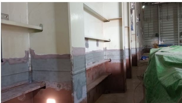
Vacuum blast in a compartment with sensitive equipment for erection joint
