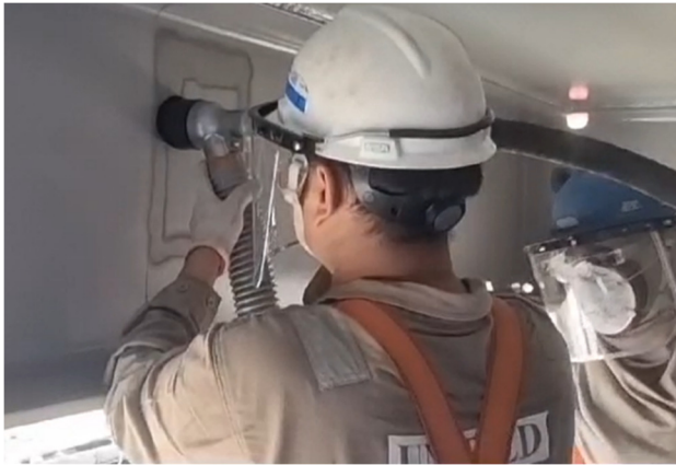
Easily to remove existing coated paint DFT 600um at 25 meter height structure (Module)
