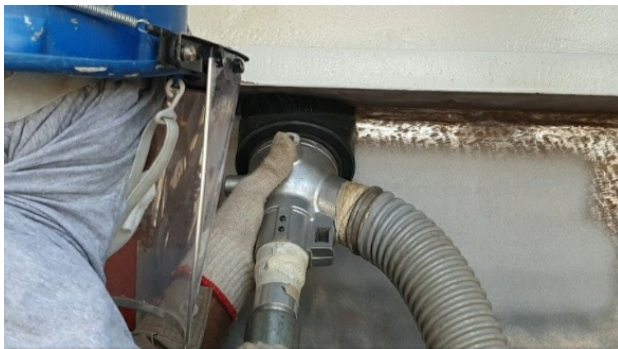
Easily to remove existing coated paint DFT 600um at 25 meter height structure (Module)
