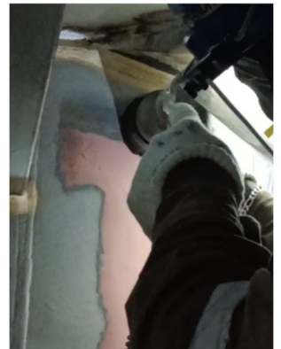
Vacuum blast at weld seam, erection joint, pipe joint, etc
